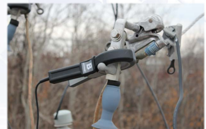
VCI-3™ in field application
